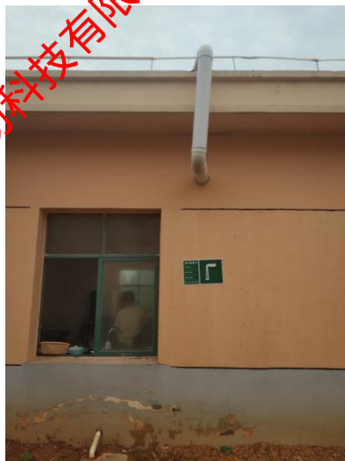
7#排气筒废气排放口标识
